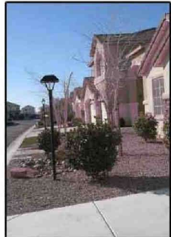
San Marino Circle H.O.A. 135 Gas Light Replacement (in process)
